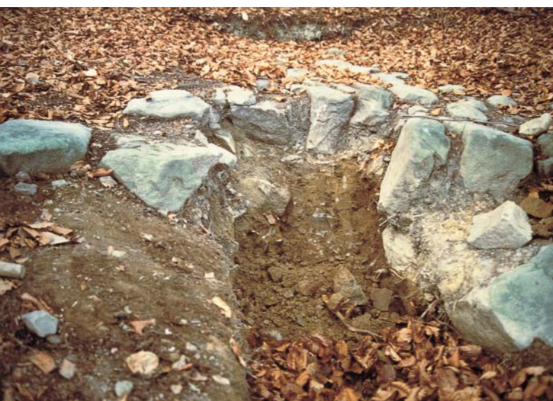
Mount Poggiaccio (site C/3): the excavation highlighted the section of the road. The paving stones came from nearby quarries. The narrower part of the stones faced downwards so that they were more solidly embedded in the layer of glarium and offered better surface resistance to the knocks they received from above.
