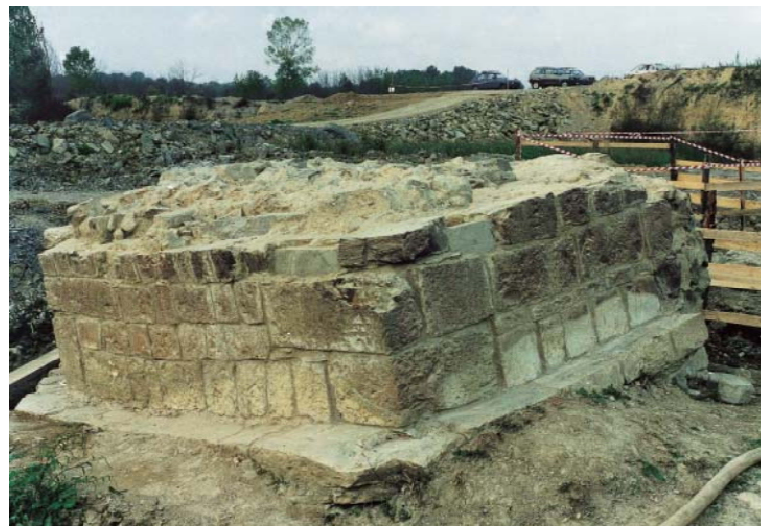
Fig. 177 – Colombaiotto bridge. The probable pier VI seen from the south on the foundation plinth.
