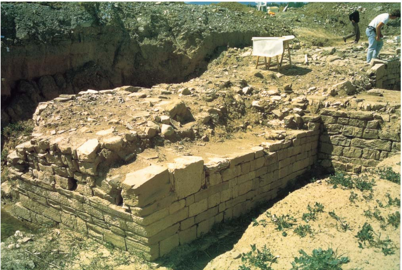
Fig. 173 – Colombaiotto bridge. Left abutment (north): downstream view of the abutment with the start of an arch and three cavities on the level of the springers.
