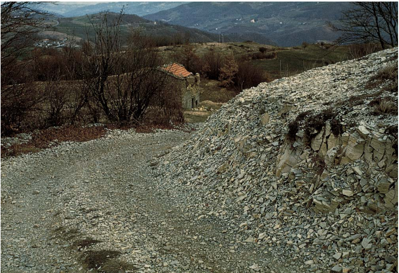
A typical example where an outcrop of limestone has been flattened to create a practical and solid roadbed. This one is 600 metres north of Predosa (archaeological zone "E") along the Roman route. It is obviously impossible to tell when the road was flattened. In the background lies the village of "Bonacca".
