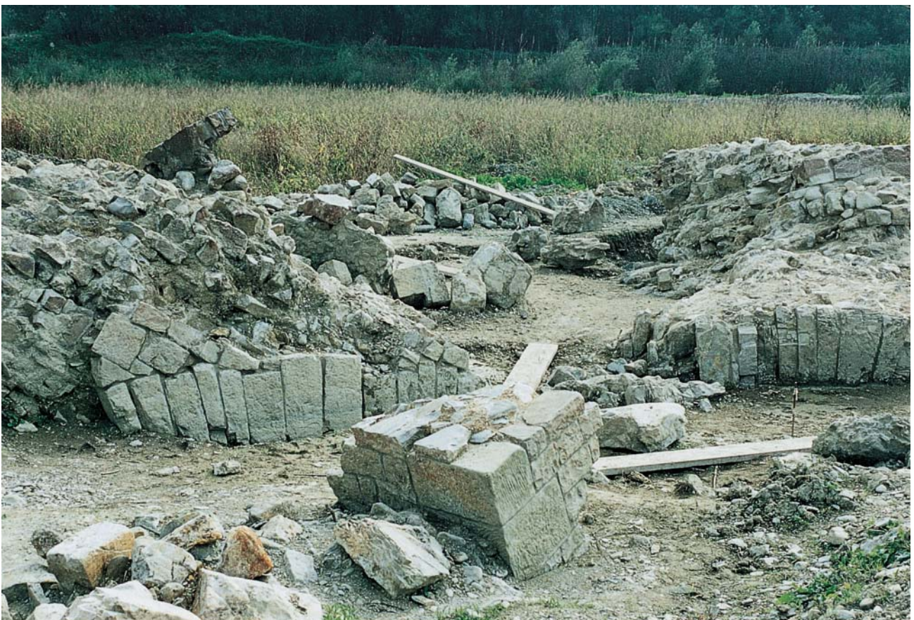
Fig. 175 – Colombaiotto bridge. The collapsed span between piers IV and V from left.
