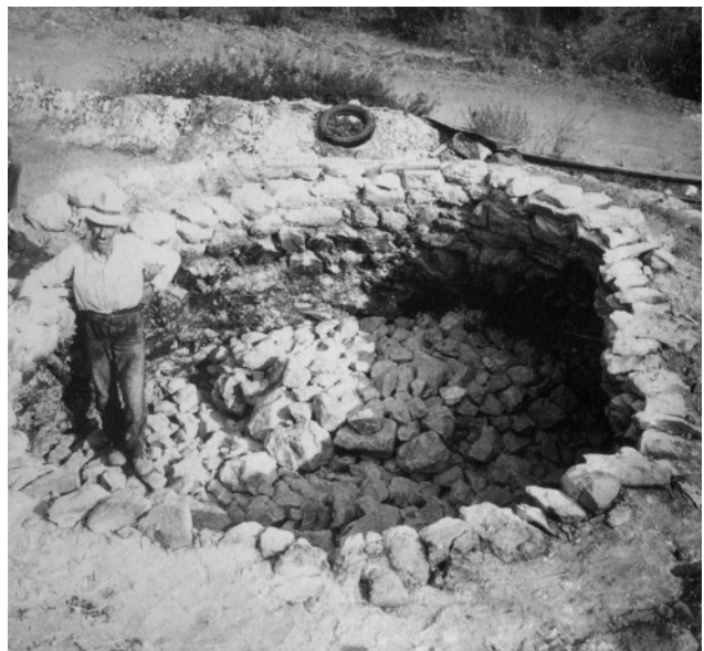
Completion of a loaded kiln near Epidauros in Greece. The same procedure has been handed down through the centuries and the similarity with the fully loaded kiln uncovered on Piana degli Ossi is striking. (From Jean Pierre Adam: “L’arte di costruire presso i Romani - materiale e tecniche” published by Longanesi e C., Milan, 1984).
