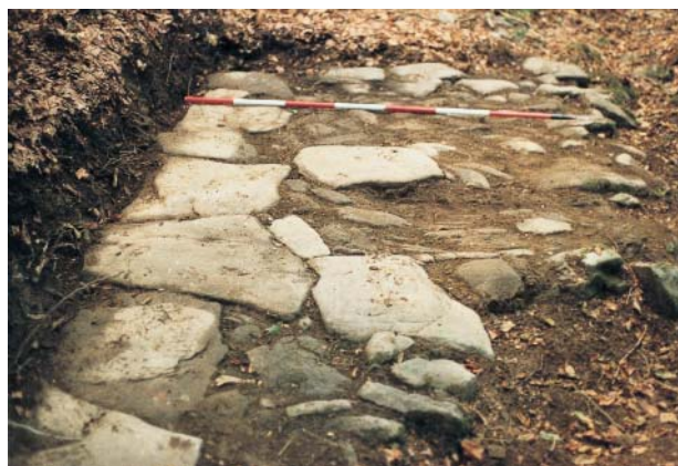
Mount Poggiaccio (site C/2-north): detail of the uphill edge of the road. Note how the stones of the original road are arranged with matching corners so that the sides match perfectly.
