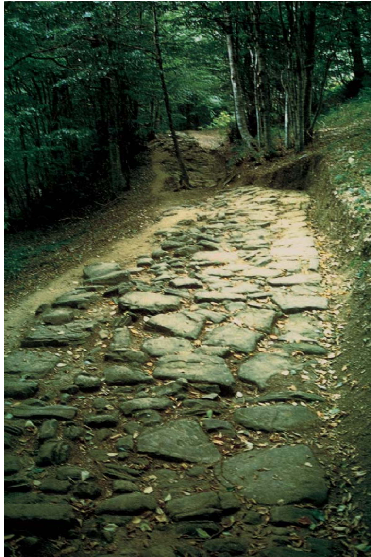
Mount Bastione (site A/1-north): the entire 19 metres of road brought to light. The part in the foreground is well preserved whereas the downhill edge of other part is uneven due to slight soil subsidence. In the background, it is possible to see the completely irregular continuation of the paving towards the left caused by a surface landslide.
