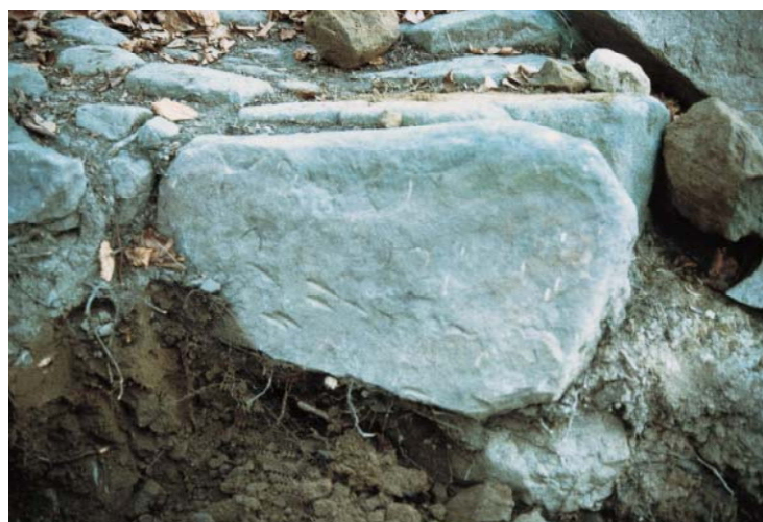
Mount Poggiaccio (site C/3): the section of paving showed that the narrow stones were laid vertically. On this stone, it is still possible to see the chiselling carried out when it was laid. We made the small white marks.
