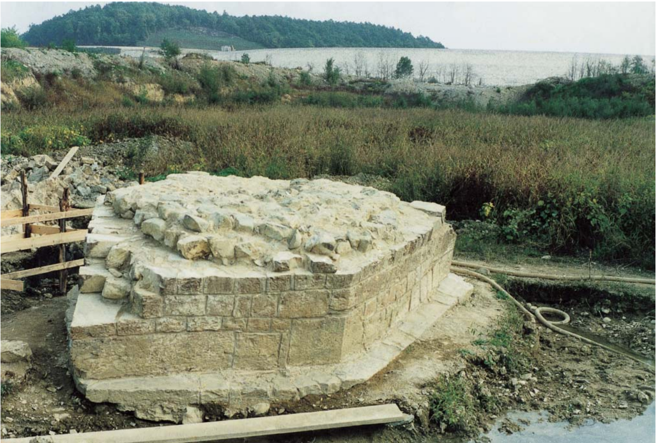
Fig. 178 – Colombaiotto bridge. The impressive rostrum (forestarling) upstream of pier VI.
