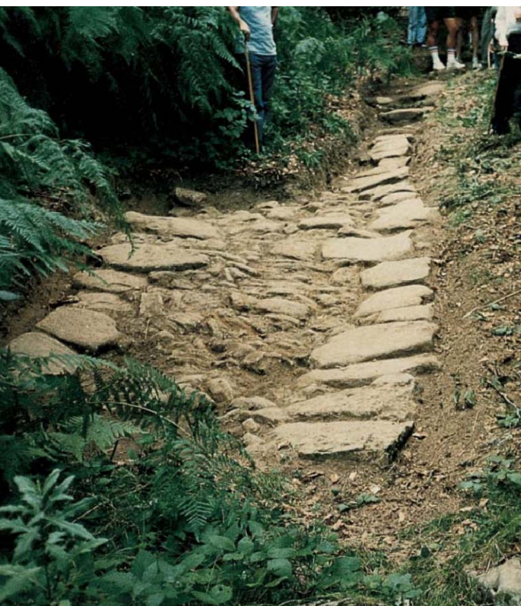
Mount Bastione (site A/4-south): along this stretch, the downhill edge of the paving (right) was also made with large sandstone blocks laid horizontally.
