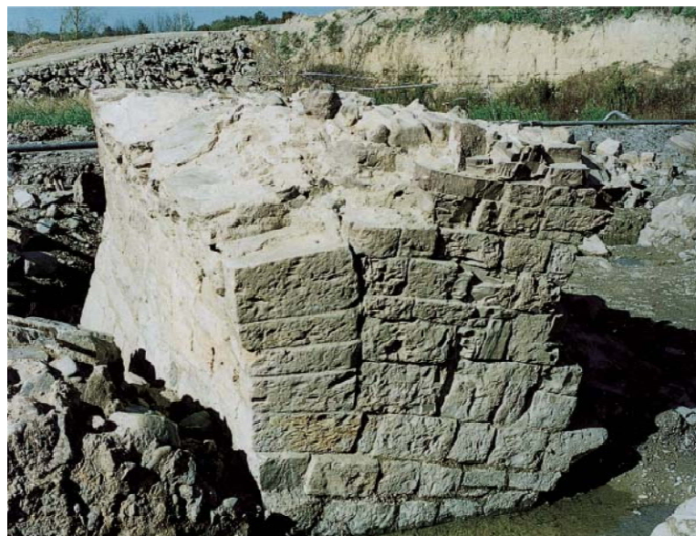
Fig. 176 – Colombaiotto bridge. Remains of courses of voussoirs still standing on the left flank of pier V downstream (they belong to the span illustrated in figure 175).
