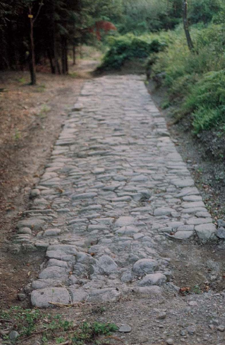
Mount Poggione (site G/4): the carriageway suddenly narrows, testifying a later repair after soil subsidence had dragged the paving downhill. The reduced 1.50 m width proves that this rough repair was carried out when the original width of the carriageway was no longer necessary.
