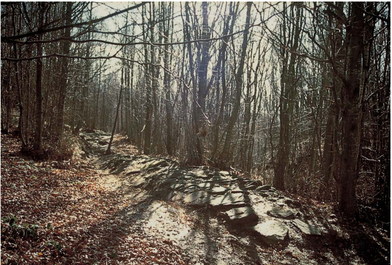
Mount Bastione (site A/2-south): the paving deformed by a surface landslide.
