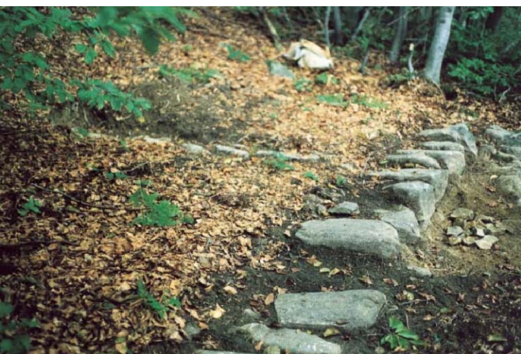
Mount Poggiaccio (site C/3): The downhill edge of the road has remained compact and in a straight line in spite of the fact that in this position, the mountain slope is very uneven.
