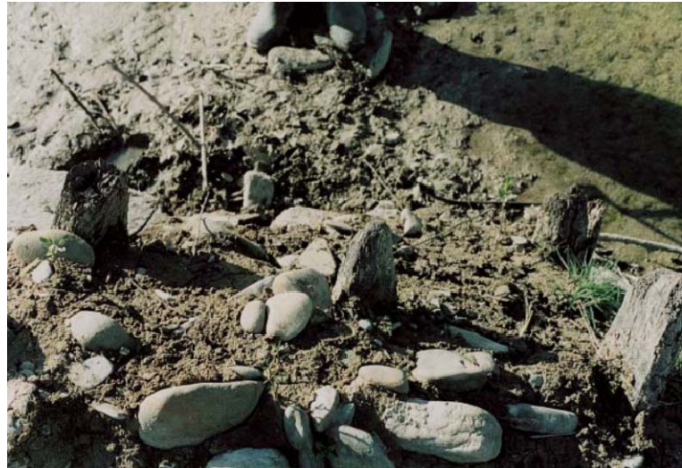
Fig. 174 – Colombaiotto bridge. Remains of probable pier II with the piles encased in its nucleus.
